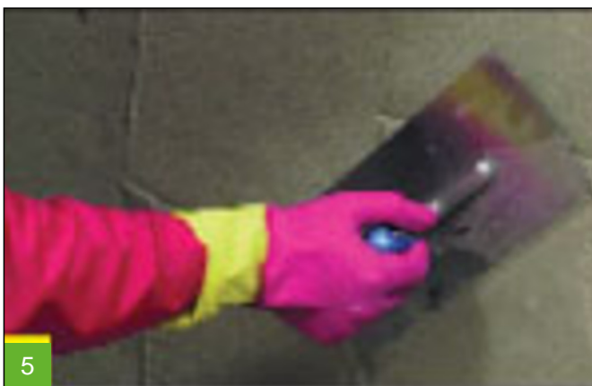
Application of the restoration render system.
