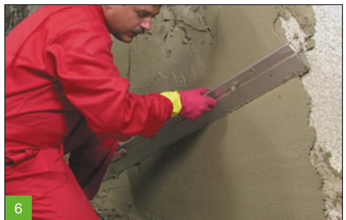
Removing any excess render and smoothing down the surface.
