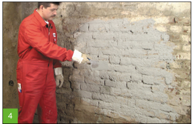
Application of the roughcast.
