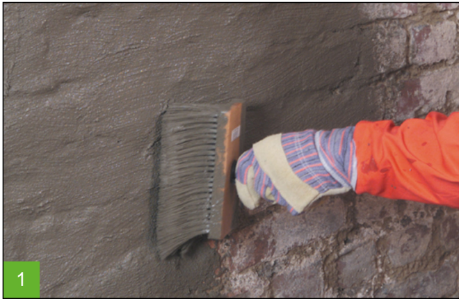
Application of the 1st layer.
