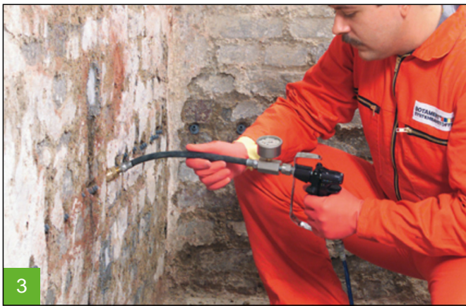
Injection with BOTAMENT &nbsp; MS 10 using pump technology
