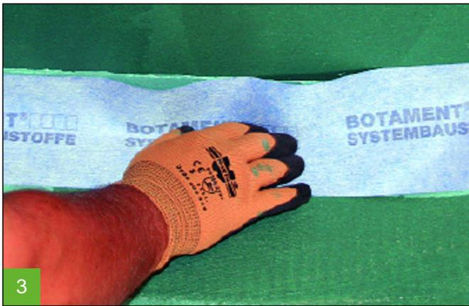
Produce the wall-floor connection with **BOTAMENT&nbsp;SB 78**.
