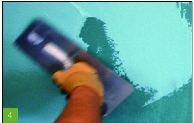
Apply the 1st and 2nd layer of **BOTAMENT&nbsp;RD 2&nbsp;THE GREEN 1**.
